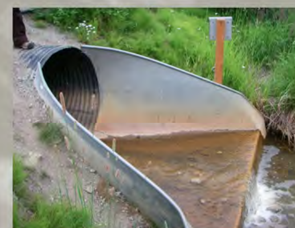
556-1 outlet from sedimentation pond
