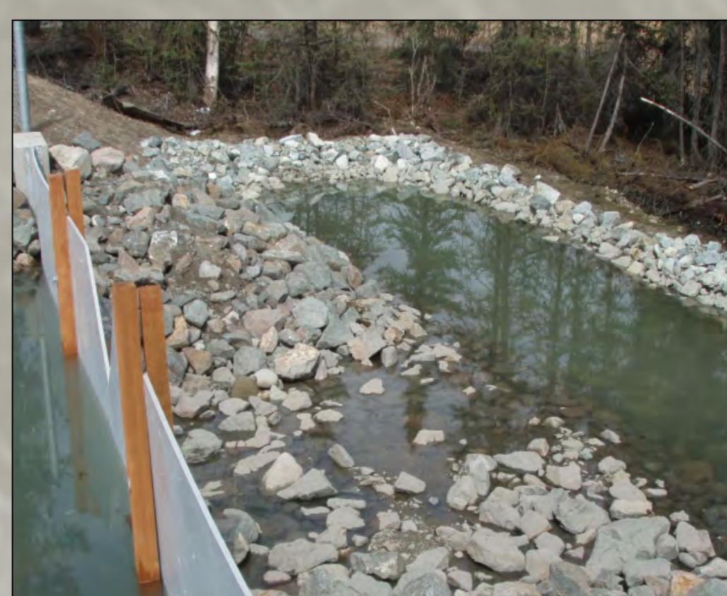
Typical settling pond located downstream from snow disposal sites.
