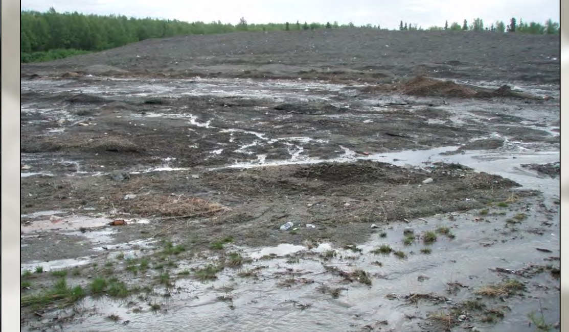
Erosion from uneven snow fill Snow collapse below deep fill
