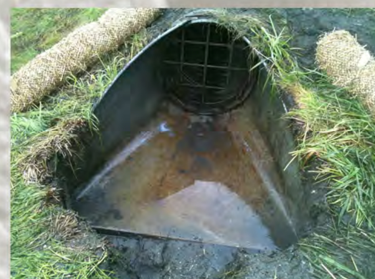
2011 Campbell Creek Outfall after cleared by MOA .
