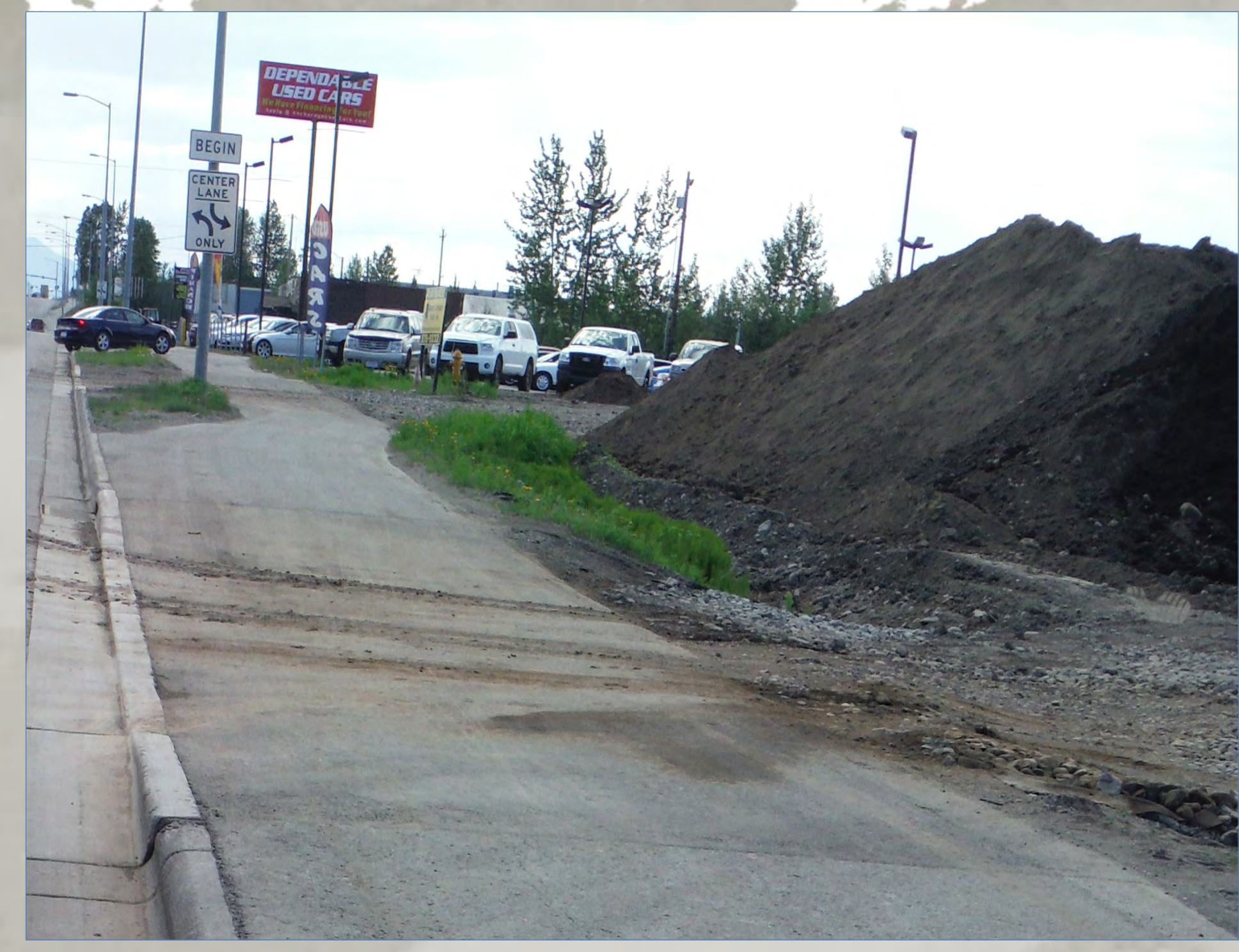
Above: A diagram illustrating the typical chronological street sediment transformations. Below: A field picture exemplifying sediment trackout from a lot to the street.
