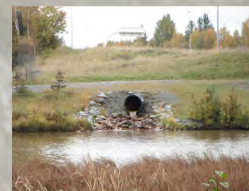
556-3 inlet to sedimentation pond
