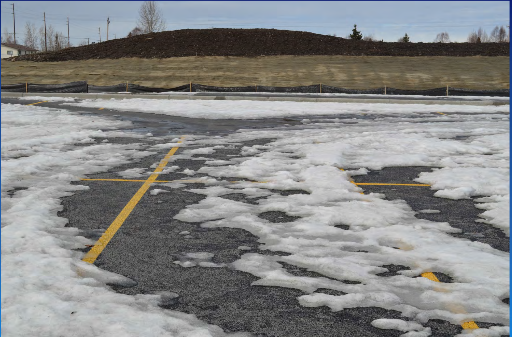
Porous Asphalt on May 1, 2013
